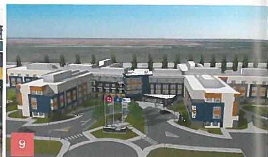
The construction schedule is only four months with factory-made precast concrete components [7]. Coloured precast concrete frames around windows give the impression of a residential-scale three-storey, rather than a four-storey building [8]. Artist rendering of the finished project. The speed of finishing the envelope using precast concrete was essential in the Alberta climate, and landscaping could begin as soon as the walls were installed, according to Peter O'Brien of Covenant Care [9].
