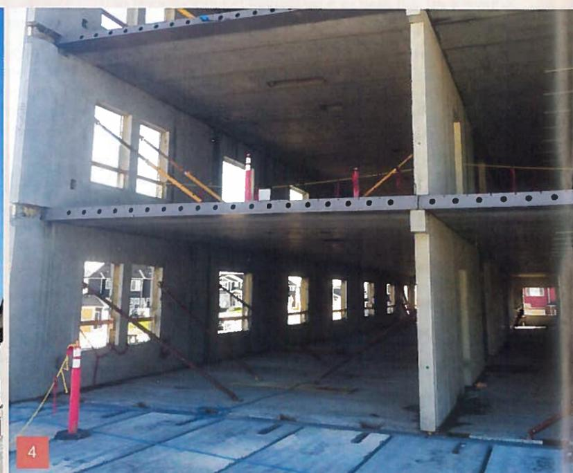
The four-storey structure, supplied by Armttec, is comprised of architectural insulated wall panels, solid interior wall panels, precast columns, stair stringers, steel Deltabeams and hollowcore floor and roof slabs supported by the exterior walls and interior beams and columns. Armttec used Tekla software for 3-D Building Information Modelling.
